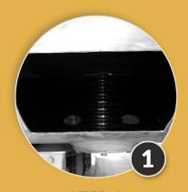
**STEP 1**Opening is cut in the enclosure
