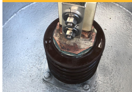
SOLUTION: CRYOGENIC CLEANING
